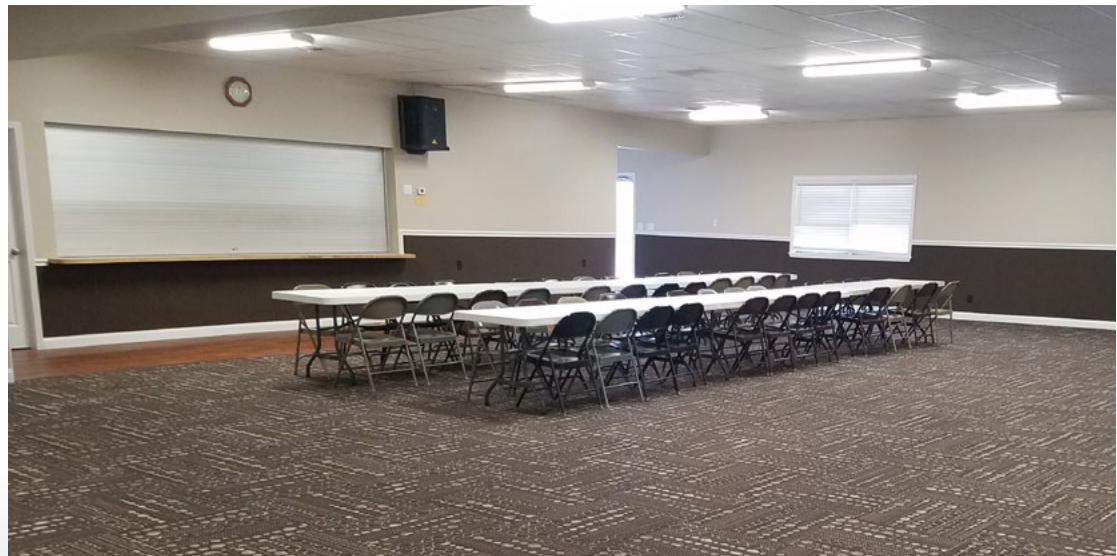
▲ The Burlington Community Club's main hall remodel included flooring, paint, woodwork, ceiling tiles and electrical outlets.
