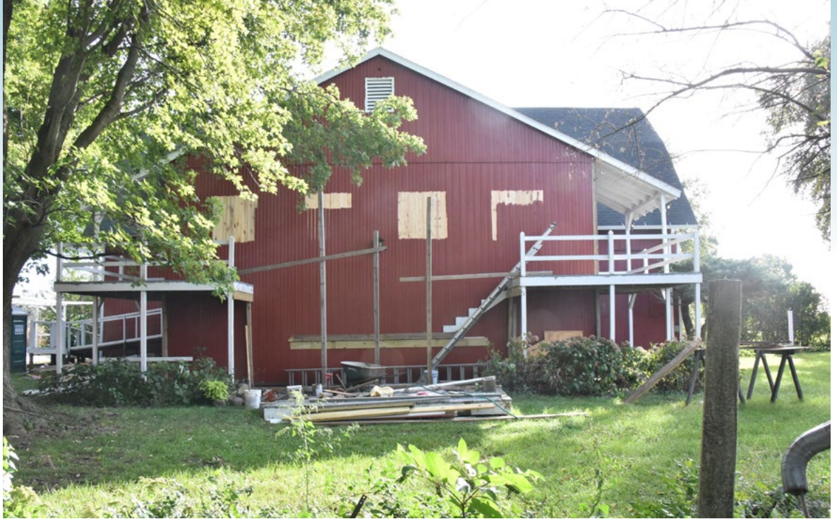
▲ The Red Barn Theatre facility received renovations and accessibility improvements.
