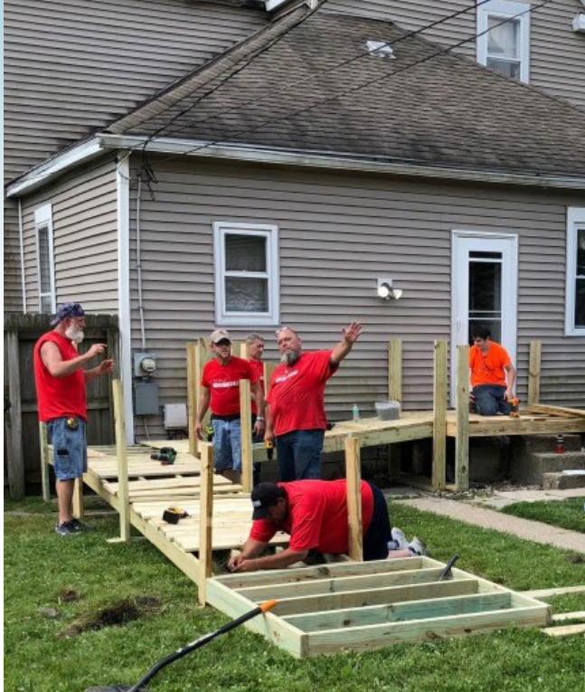
▲ Volunteers assemble a wheelchair ramp through the Servants at Work program.
